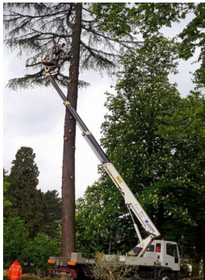
Camion Nacelle 24m
